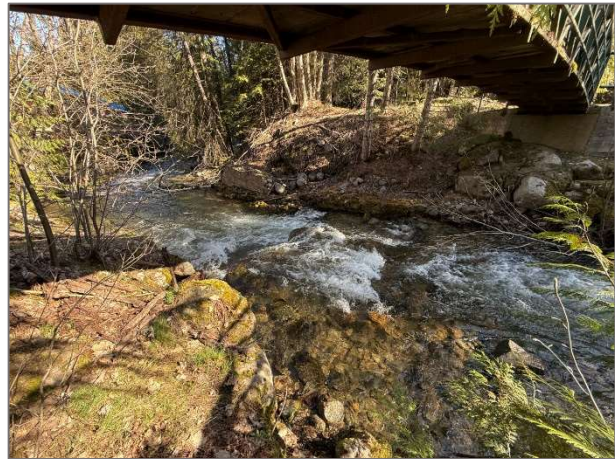
Photo 2. Springer Creek pedestrian bridge eastern abutment, April 2025.
