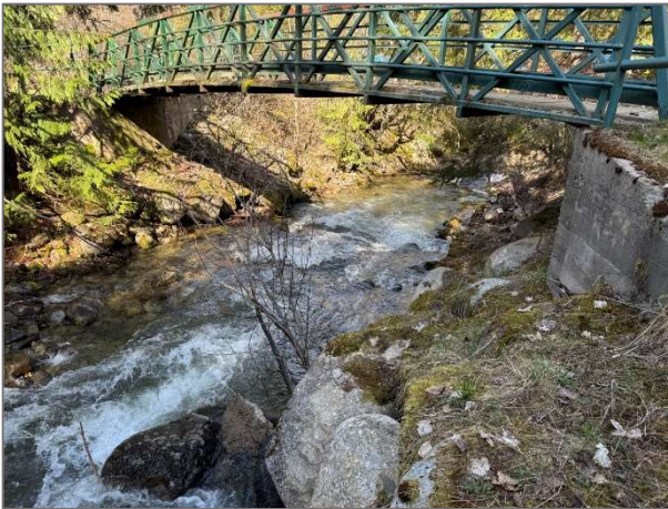
Photo 1. Springer Creek pedestrian bridge western abutment, April 2025.
