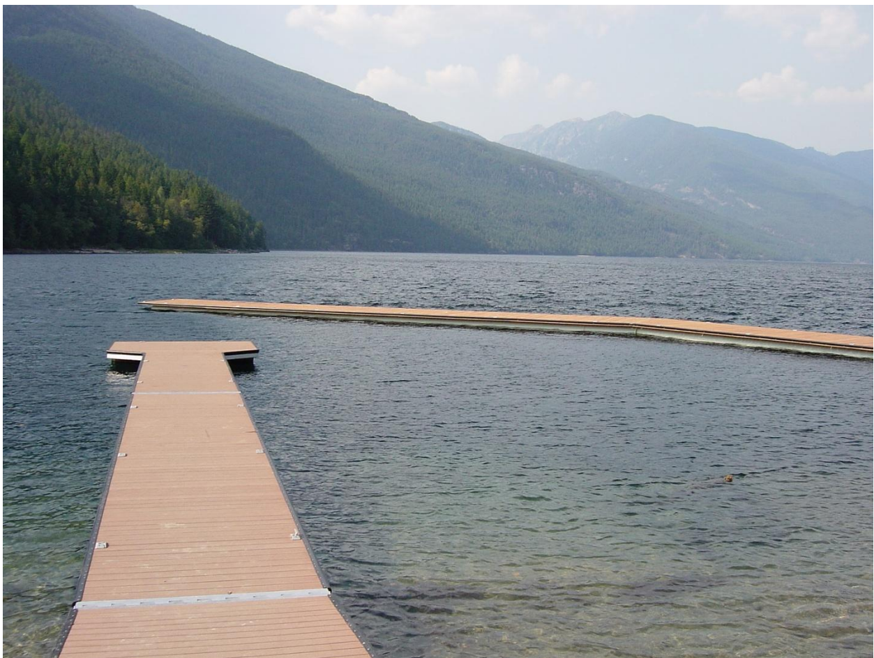
2006 – BREAKWATER AND BOAT LAUNCH DOCK
