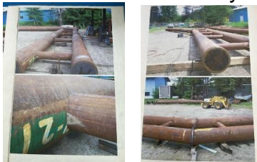
CONSTRUCTION OF BREAKWATER 2006
